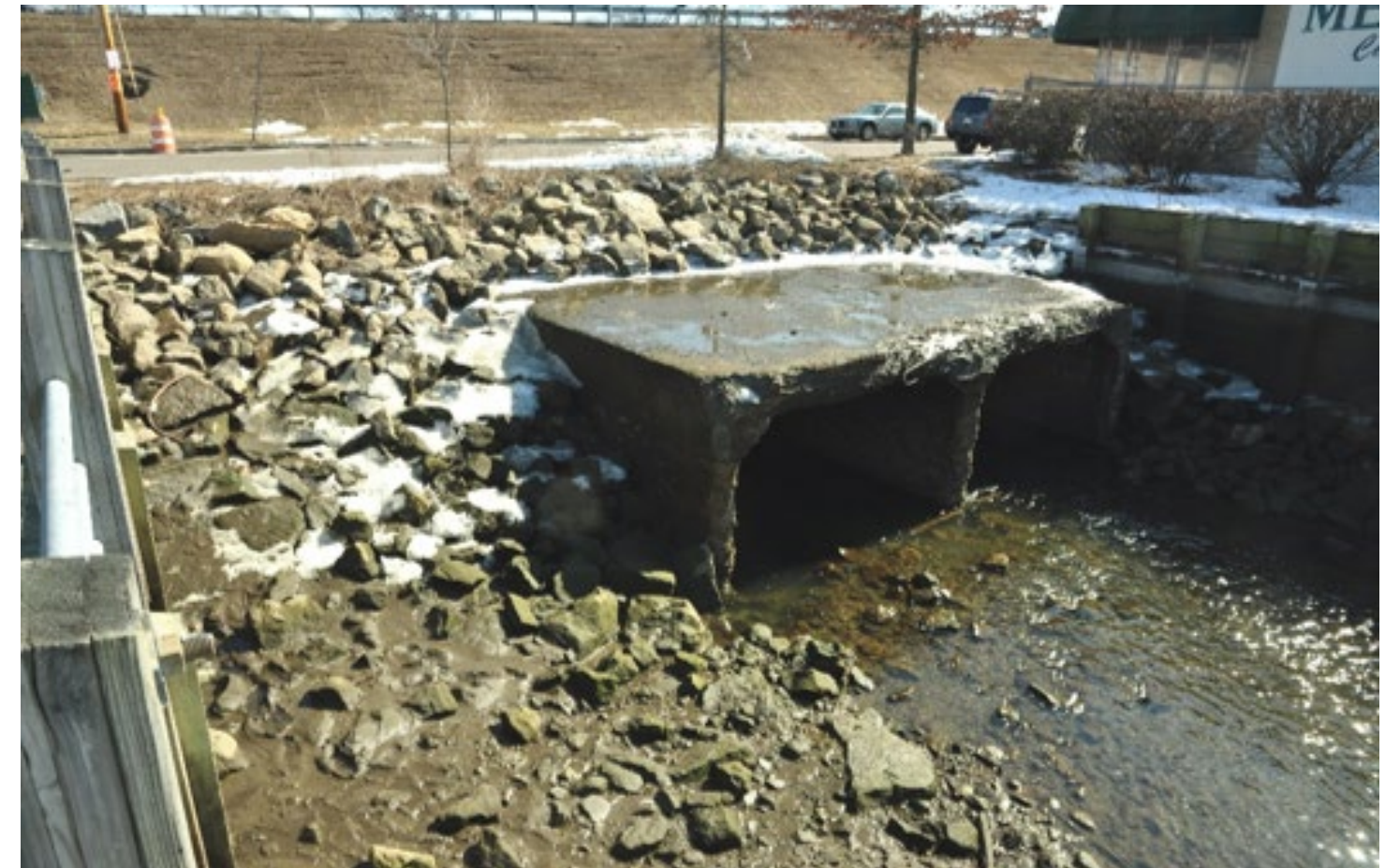
West Headwall – Looking NE
