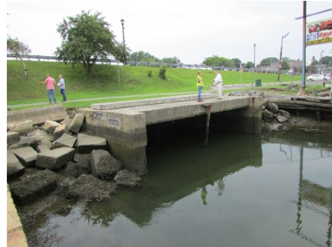
Downstream Face of Culvert with Gate Remnants
