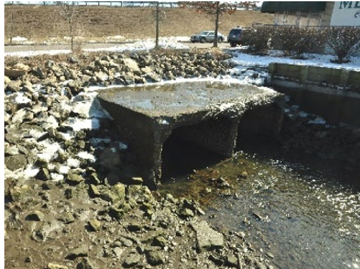
Upstream Face of Culvert at Low Tide
