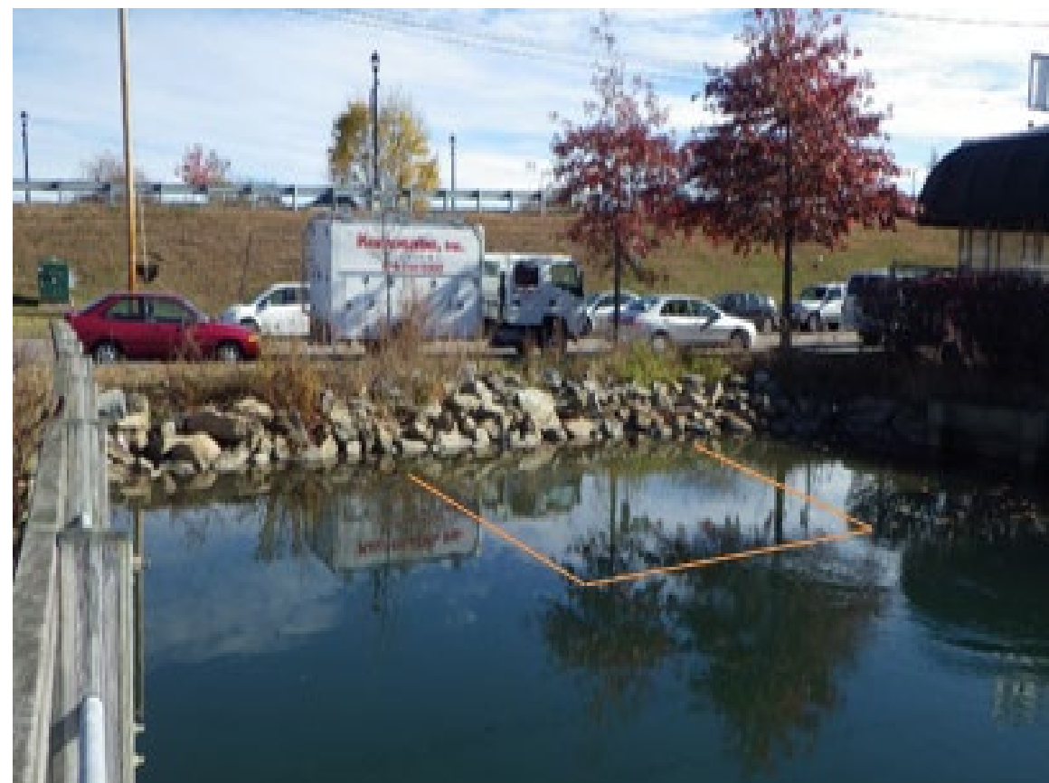
Upstream Face of Culvert at High Tide
